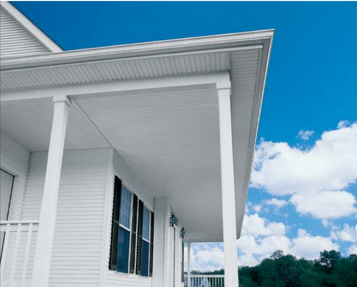
Beaded detail enhances the charm of porch ceiling and overhang installations.
